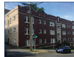
$28,300,000 Multifamily Houston, TX 3 year term and extensions Acquisition, renovation and lease-up
