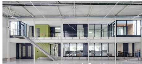
$28,680,000 Vacant Life Science Building Menlo Park, CA
